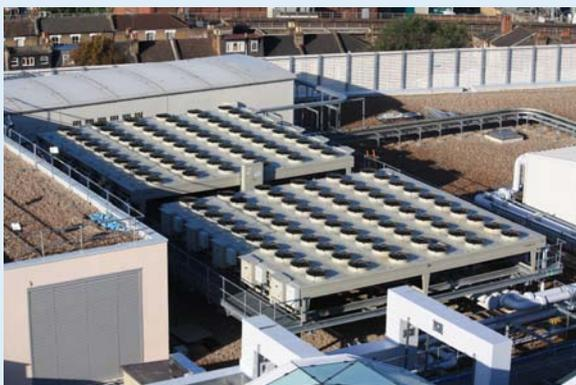
61 Güntner GFH drycoolers ensure low-noise and energy-efficient operation at Westfield London.
