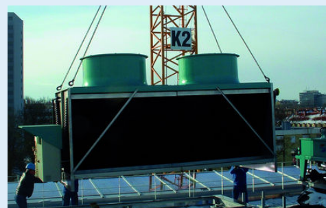
Hybrid coolers of Jäggi/Güntner: Ideal for the application in clinical areas due to the absence of legionella and the emission protection suitable for clinics. Photo above: 2 HTK, model 1.8-52-2S-B6-BU-SX3.
