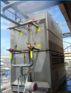
▲ Two Güntner ECOSSE evaporative condensers dissipate the waste heat of the NH<sub>3</sub> compressors into the ambient air.
