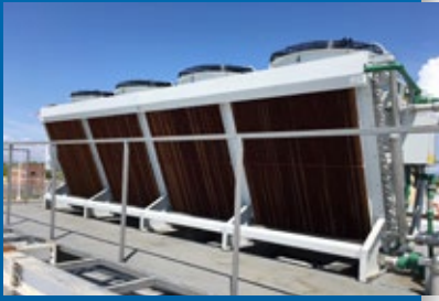
▲ The Güntner gas cooler V-SHAPE Vario GFW is equipped with the Güntner Motor Management GMM for the speed control of the EC fans and with the Güntner Hydro Management GHM that controls the water supply.
