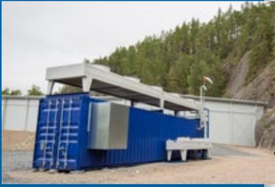
▲ The waste heat of the secondary circuits is dissipated to the environment via a Güntner dry cooler FLAT Compact GFH (new series: GCHC) equipped with EC fans and GMM.
