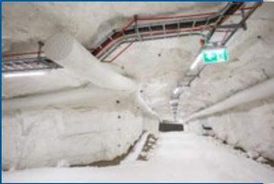
▲ The cold as well as the supply air is routed via textile socks, resulting in a total length of 2.4 km of air textile socks installed in the mountain. Depending on the distance to the air conditioning unit, the conditioned air is distributed either via ten Güntner CUBIC Vario air coolers type GGHN (new series: GACV) with streamer (at the entry area), or via textile socks (inside the mountain).
