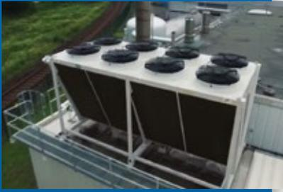
▲ In winter, the free cooling function of the GFD-type Güntner V-SHAPE Vario achieves impressive savings in terms of heat dissipation from the injection moulding plant.
