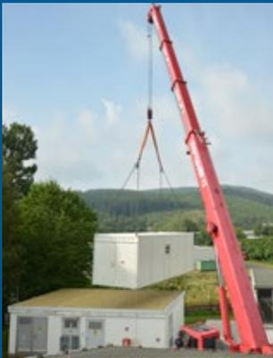
▲ As the boiler room was too small to house seven adsorption chillers, the goal was to place all the cooling equipment in one container, which also had to have special dimensions as it had to be installed in a gap between two buildings.
