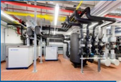
▲ The machine room with five adsorption chillers provides air conditioning at the Miele plant in Bünde.
